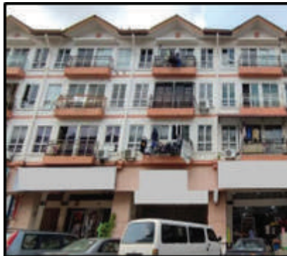
Rajah 15: Rumah Pangsapuri ( Apartment )
